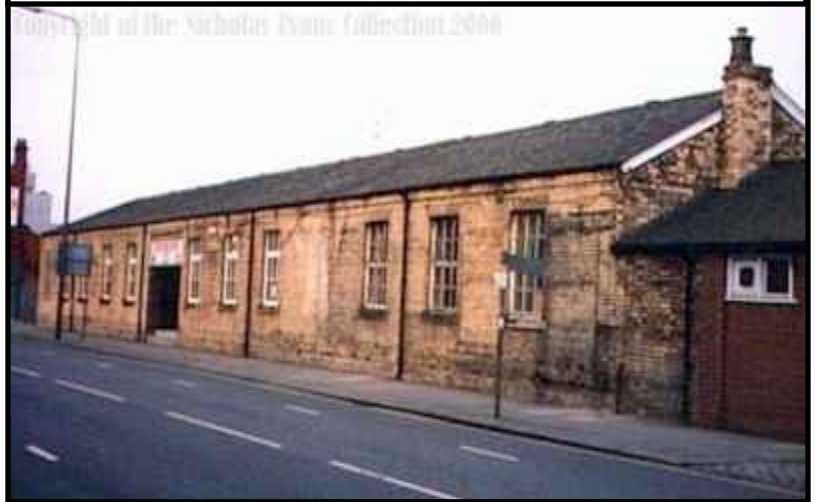
Photo of the Emigrant Waiting Room of the North Eastern Railway Company at the Hull Paragon Railway Station. The waiting room was built for Scandinavian immigrants passing through Hull in 1871, and then extended in 1882.
